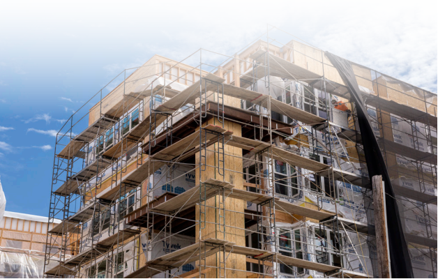
First Community Housing employed modular components to accelerate the building process for the Second Street Studios (shown here under construction). The project is one of the first to receive funding from Measure A and will provide 135 permanent, supportive homes for previously homeless individuals. Photo: Jeffrey Peters
